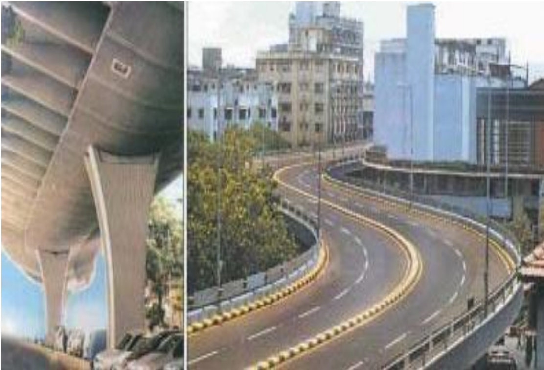
Fig 34: Flyover at Mumbai where high strength, high performance concrete 75 MPa was used for the first time in India (2002)
