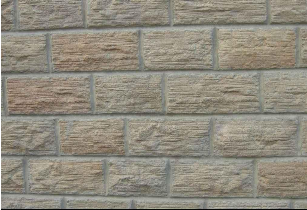
Course Rubble Stone Masonry Wall
