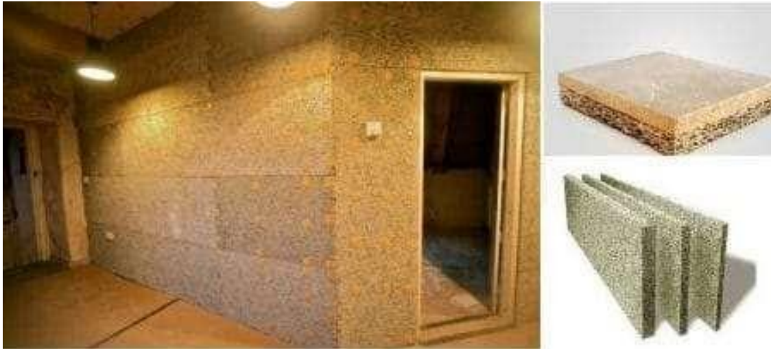
Fig.15: Wood-wool partition wall
