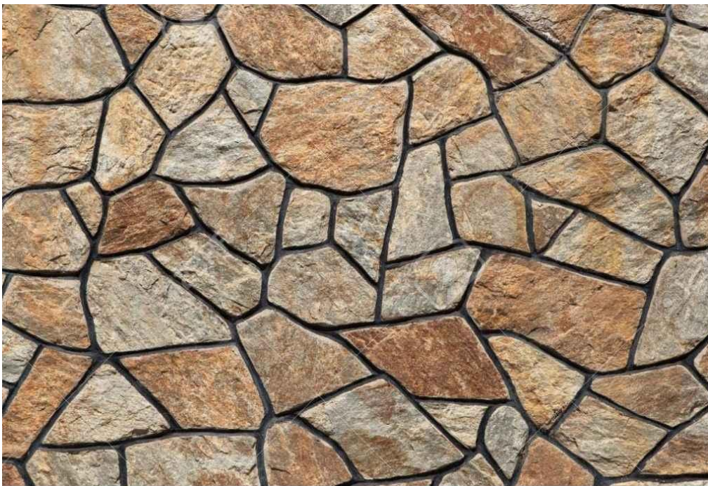
Random Rubble Stone Masonry Wall
